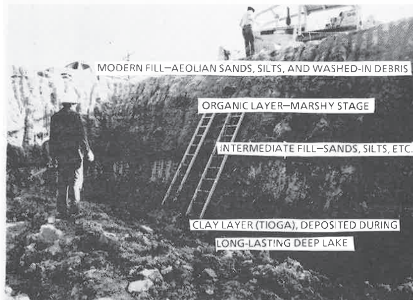
PHOTO 4. Construction Pit on China Lake Playa. This photo shows the climatic and geologic changes through stratigraphy since the Tioga phase of the Pleistocene.
